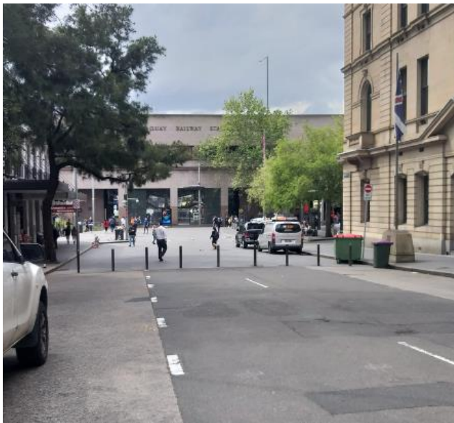
Figure 7: Loftus Street terminus looking north (Source GYDE Consulting September 2022)
