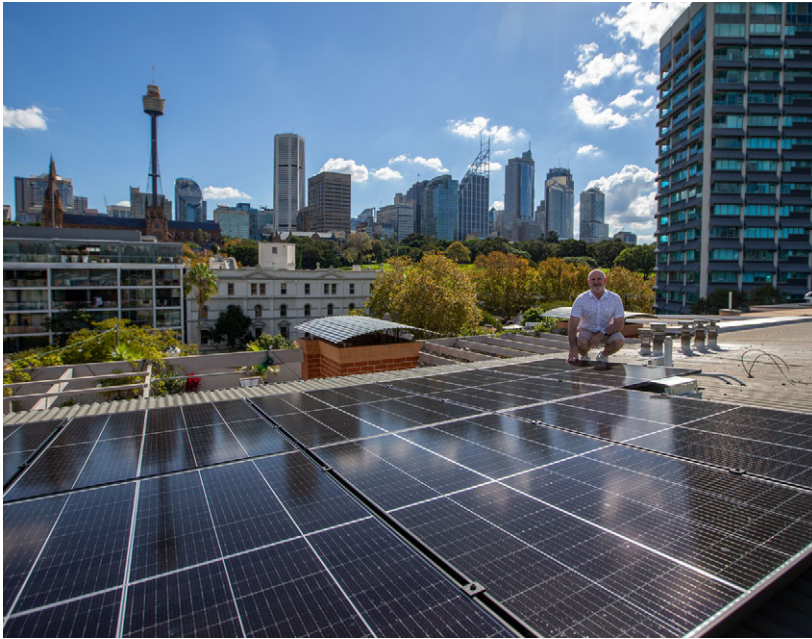
Rooftop solar on The Galleria apartment building
