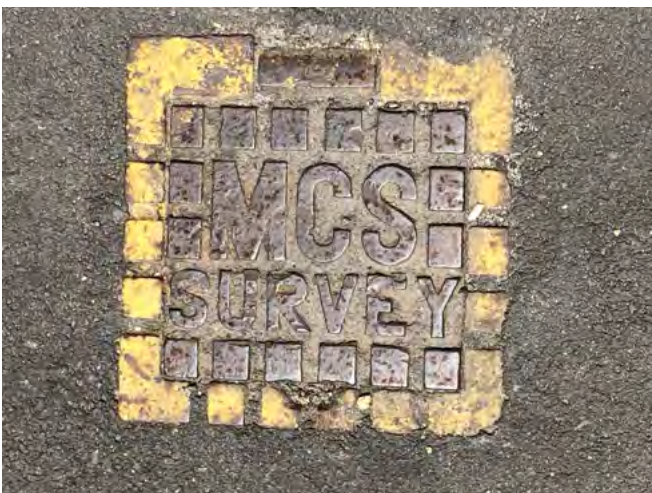
Figure 5a - Permanent mark cover box
