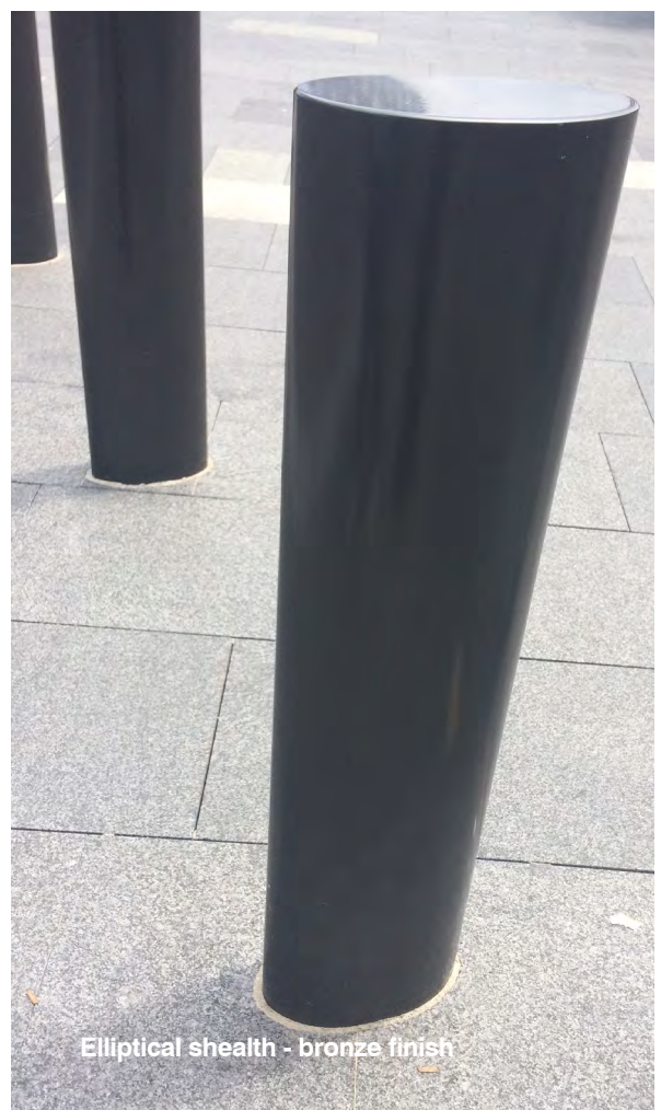
City standard bronze sheath to house structural component ( indicative only under design development)
