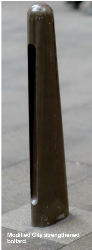
City standard bronze sheath to house structural component ( indicative only under design development)
