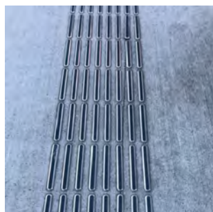
Stainless steel TGSI - directional
