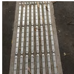
Stainless Steel TGSi directions
