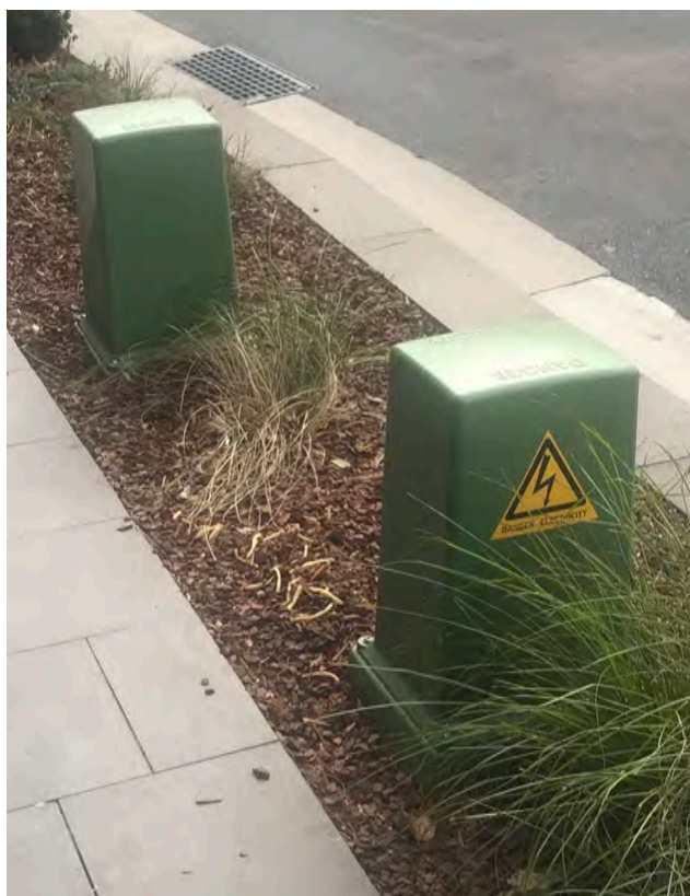
Electricity surface kiosk pillar
