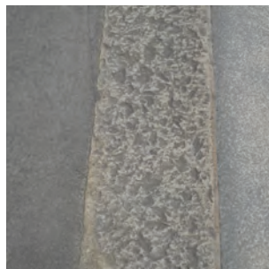
Trachyte retain and reuse existing stone kerb as directed by the City
