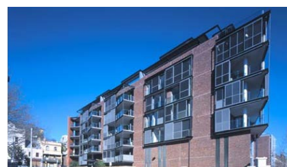
Figure 22: Walsh Bay Apartments (Mirvac) Example building design showing setback upper storeys, defined street wall and articulated façade.
