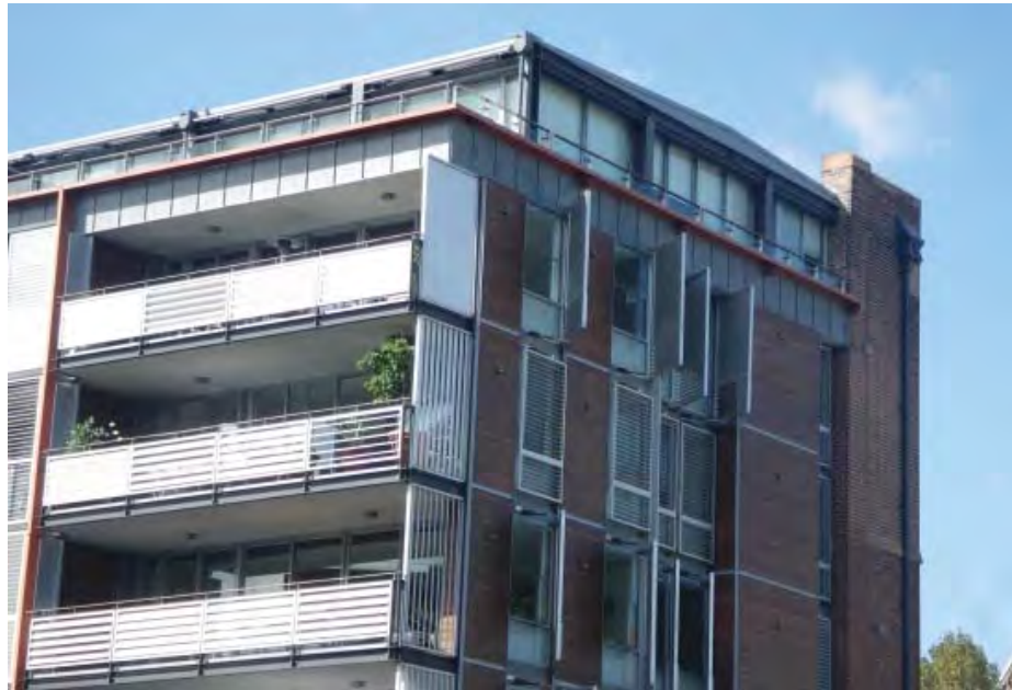
Figure 5.127 Example of good building articulation, Walsh Bay
