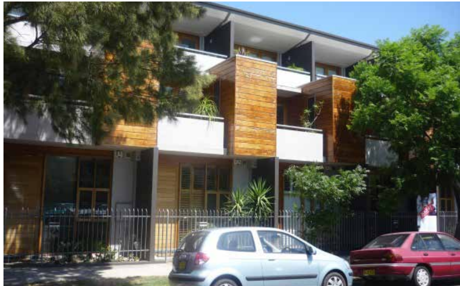
Figure 5.153 Example of developments that use a range of building materials, Alexandria
