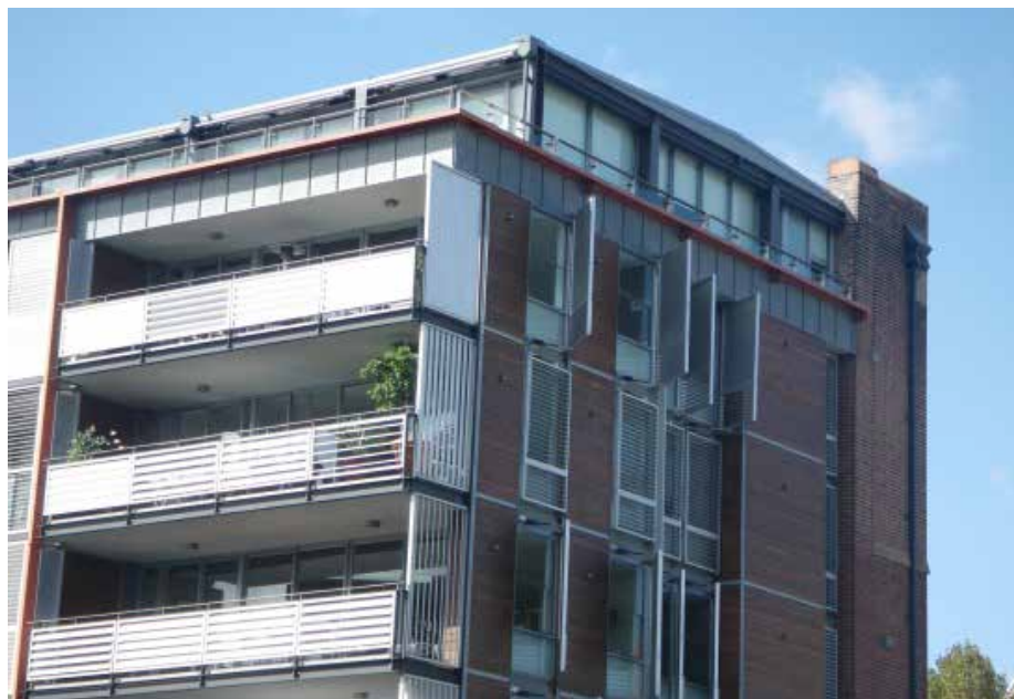
Figure 5.142 Example of good building articulation, Walsh Bay
