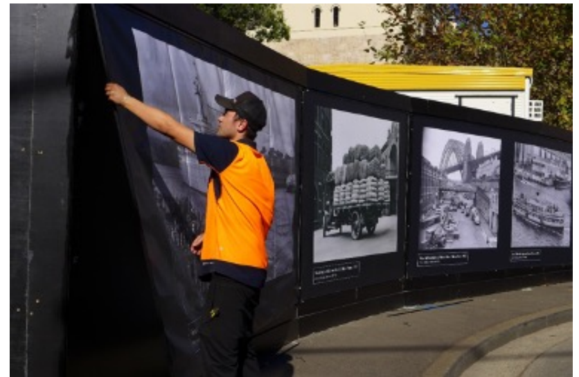
Installing printed vinyl on a 'Type-A' hoarding. Black powder-coated sail track must be used. Photo by City of Sydney.
