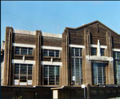
Art Deco style brick building enveloping the Waterloo Water Pumping Station
