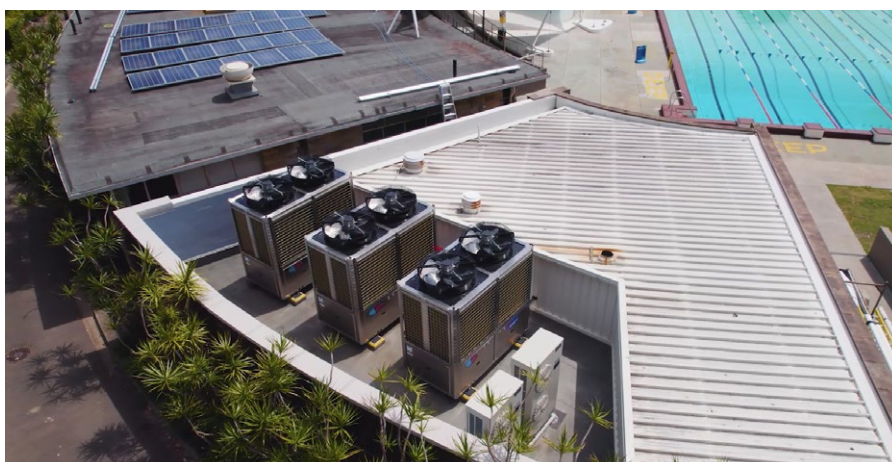
Electric heat pumps replacing gas at Victoria Park Pool. Credit: Supplied by Image Air
