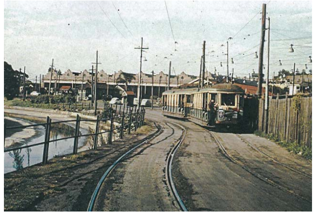
'O' type coupled set of trams Nos.1462 and 1359 on the road to Rozelle Tram Depot, 1958, showing historic fence, and extensive pole gantries for overhead power.
