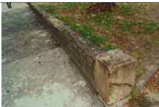
Fig. LH5 Close-up view of the dwarf sandstone wall with coping stone and squared driveway entrance block, Chamlers St. boundary
