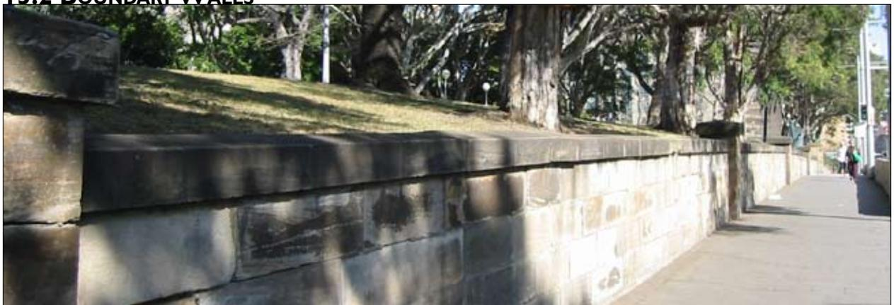
New boundary walling to match existing raked sandstone block walls, piers and capping stones.
