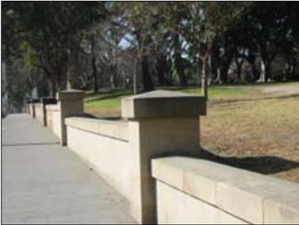
*Maintaining consistency and continuity in established design language is important. Stepped walls have recently been introduced on the Park Street boundary where all existing historic wall copes slope with the ground plane.*
