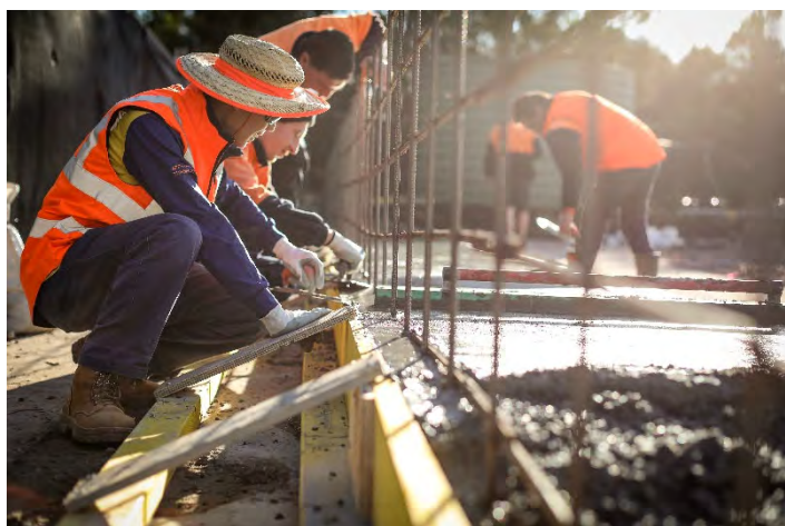
Image 2. City of Sydney maintenance crew construction concrete footpath at Sydney Park 2019
