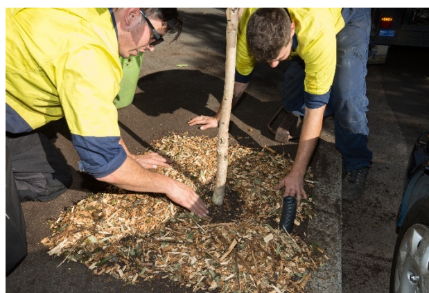
Images above show tree being planted, watering coil being installed and mulched. City of Sydney 2016.
