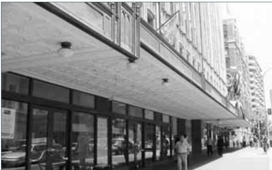
Figure 1 Awnings define and shelter pedestrian space (Castlereagh Street).
