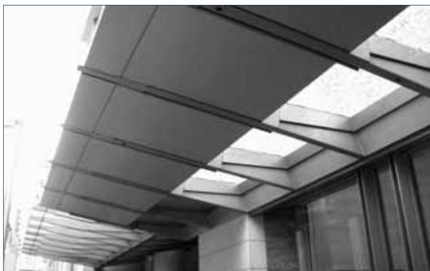
Figure 4 Contemporary Awning Design at 400 George Street, 1999.
