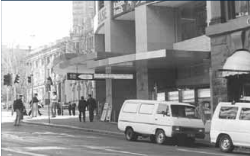
Figure 9 The awning steps with the topography and highlights the corner location (cnr Bridge and George Streets) responding to the streetscape.
