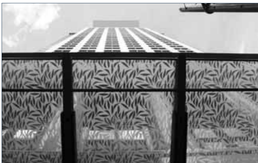
Figure 16 Glass in awnings is to be coloured either clear or very lightly tinted, and patterned to mask dirt. At significant places along awnings, such as at this major building entry pictured, additional glass may also be appropriate.
